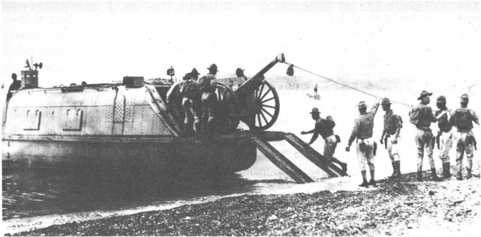
AN EARLY VERSION OF THE LANDING CRAFT used in World War II which resulted from joint Navy-Marine Corps experiments in the 1920's and 30's. (USMC 515227)
