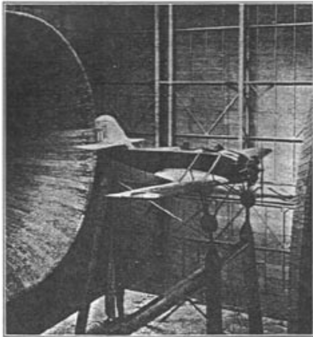
FIGURE 1.—The McDonnell airplane with large fillet in full-scale wind tunnel.
