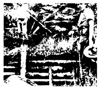
Photo credit: us Forest Service A catch dam, constructed from local materials, is used i n the gully to halt further soil erosion
