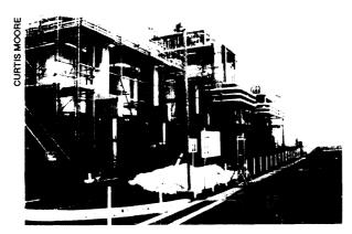
Tokyo Electric Power Company's 11 megawatt phosphoric acid fuel cell is the largest fuel cell installation in the world. Most of Japan's environmental R&D concentrates on improving energy technologies.
