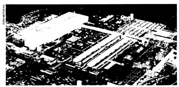
U.S. automakers spend large sums to build and operate facilities to control painting emissions. Ford estimates that it has spent between \$150 to \$180 million to build its recent paint shops, of which \$20 to \$40 million is to control pollution. The paint shop (on the left) of this Ford truck plant in Virginia is larger than the assembly line building on the right.
