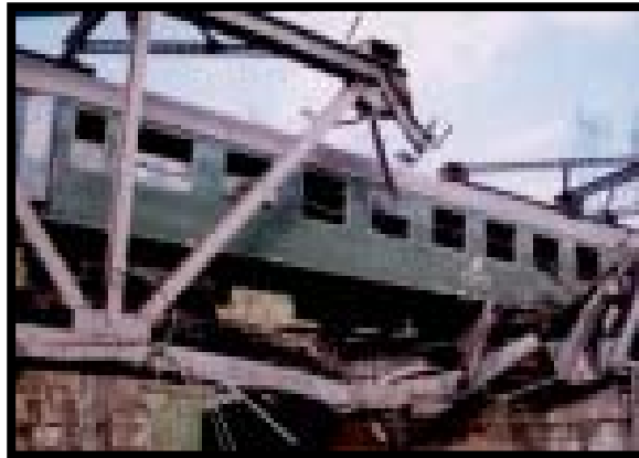
Figure 7-24. Example of a damaged rail transportation system.
