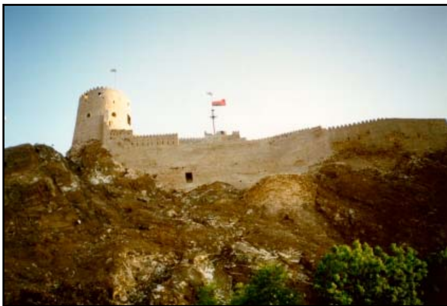
Figure 2-9. Permanent or fixed fortifications.
