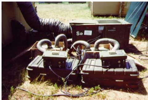
CB hardened environmental control unit with M28 chemical filters and blowers
