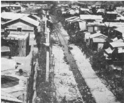
Perimeter of Nha Trang Air Base, separated from the city by two concertina fences on either side of a drainage ditch
