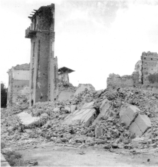
Bombing raids on the airfield at Ciampino reduced buildings to rubble ( left ). Some had their steel skeletons exposed ( upper left ). Wrecked aircraft littered the field ( upper right ).
