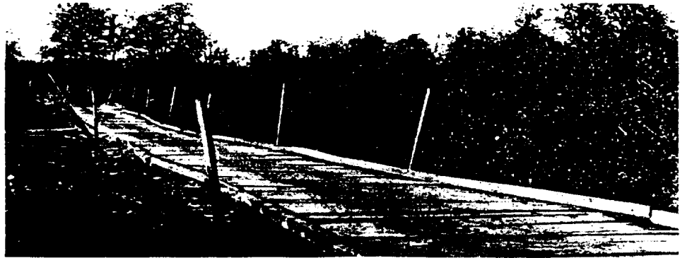
Section of Avocourt-Montfaucon Road Showing Plank Construction
