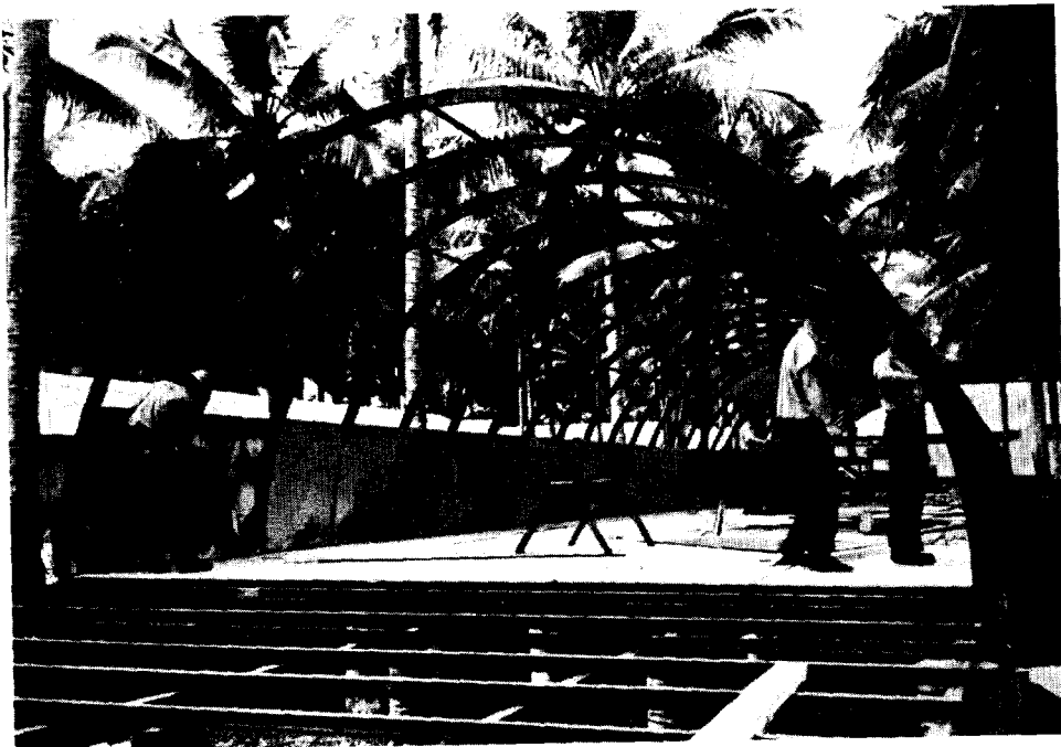
FIGURE 147.—Anatomy of a quonset hut; erecting the ribs.
