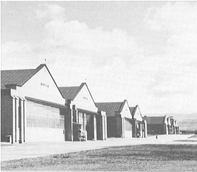
Above, engineering buildings and parachute shop; left, the flight line; and, below, the fire station at Wheeler in 1940. (Vincent T. Ryan)
