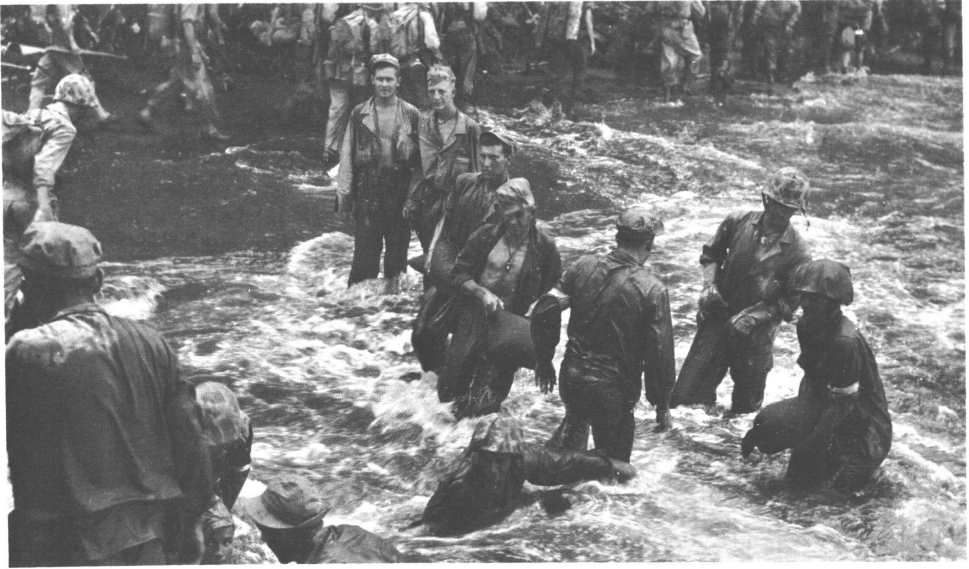
SHORE PARTY MARINES struggle to build a sandbag ramp for LSTs in the surf at Cape Gloucester's Yellow Beaches. (USMC 68999)
