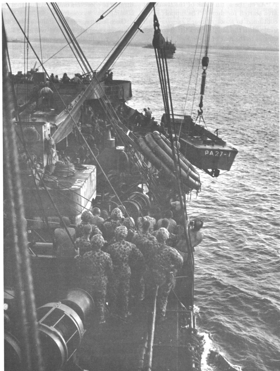
LANDING CRAFT is lowered over the side of the APA George Clymer on D-Day at Bougainville while Marines watch in the foreground. (USN 80-G-55810)
