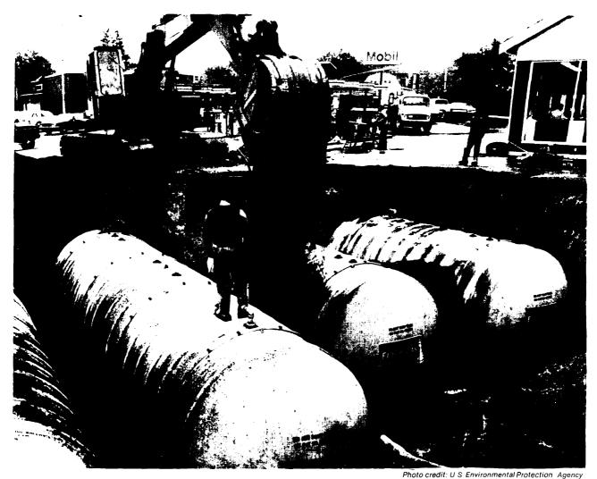
Voluntary replacement of underground gasoline storage tanks is one technique that many States rely on to prevent groundwater contamination.
