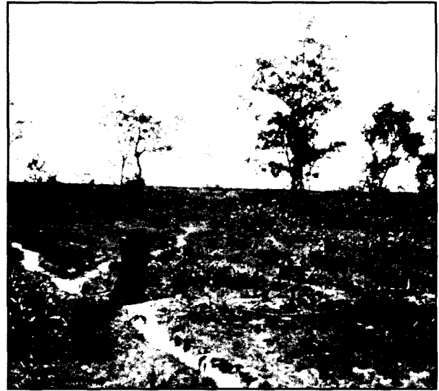
(U) Udorn site before construction started in 1965
